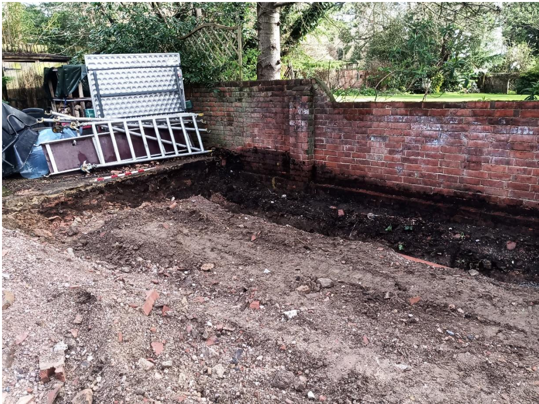
Plate 4. Foundation raft ground reduction (looking NW)
